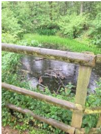
Photo Wooden Fencing
